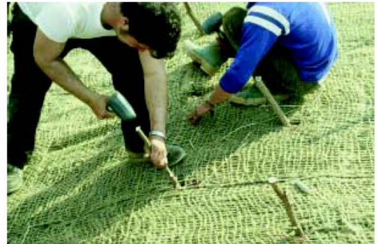
Live staking. Robbin Sotir & Associates
